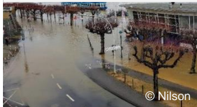
High water levels
